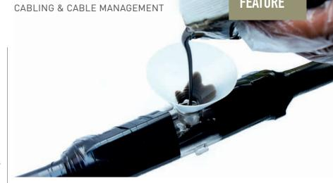
Resin cable joints are an essential for contractors who are repairing damaged cables
